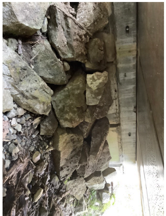
Left Bank Abutment when facing downstream
