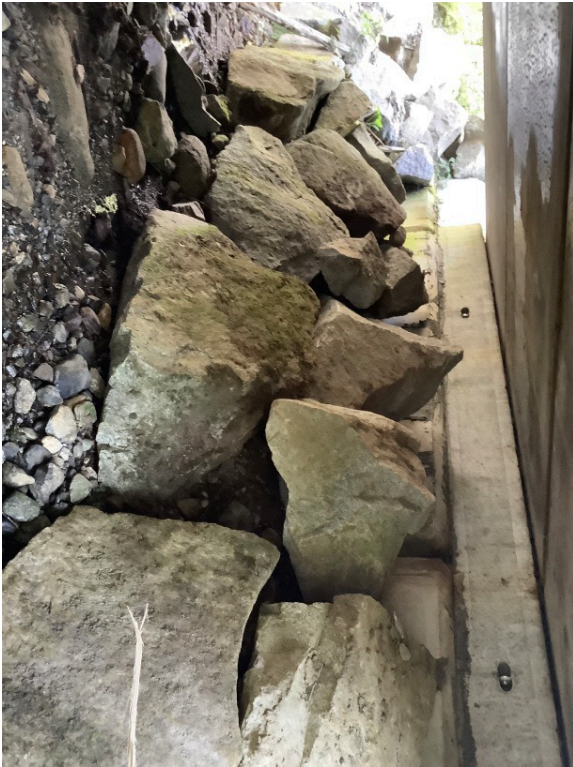
Right Bank Abutment when facing downstream
